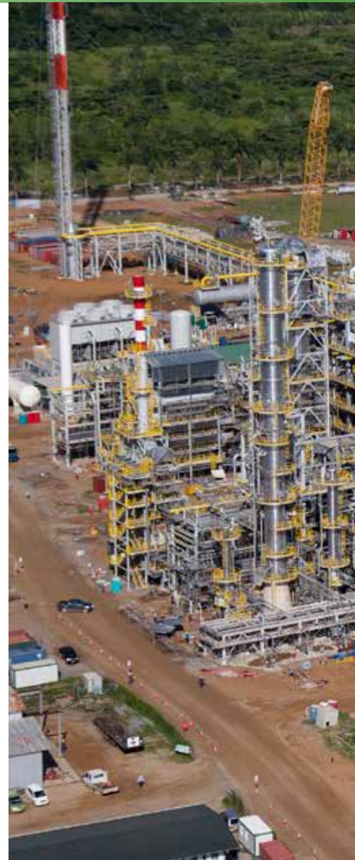
De raffinaderij vanuit de lucht. An aerial view of the refinery.
