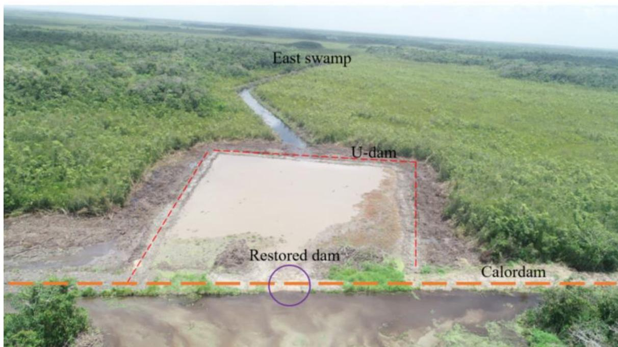
**Figure 3: Overview constructed U-dam and Calor Canal (ILACO, 2021)**
