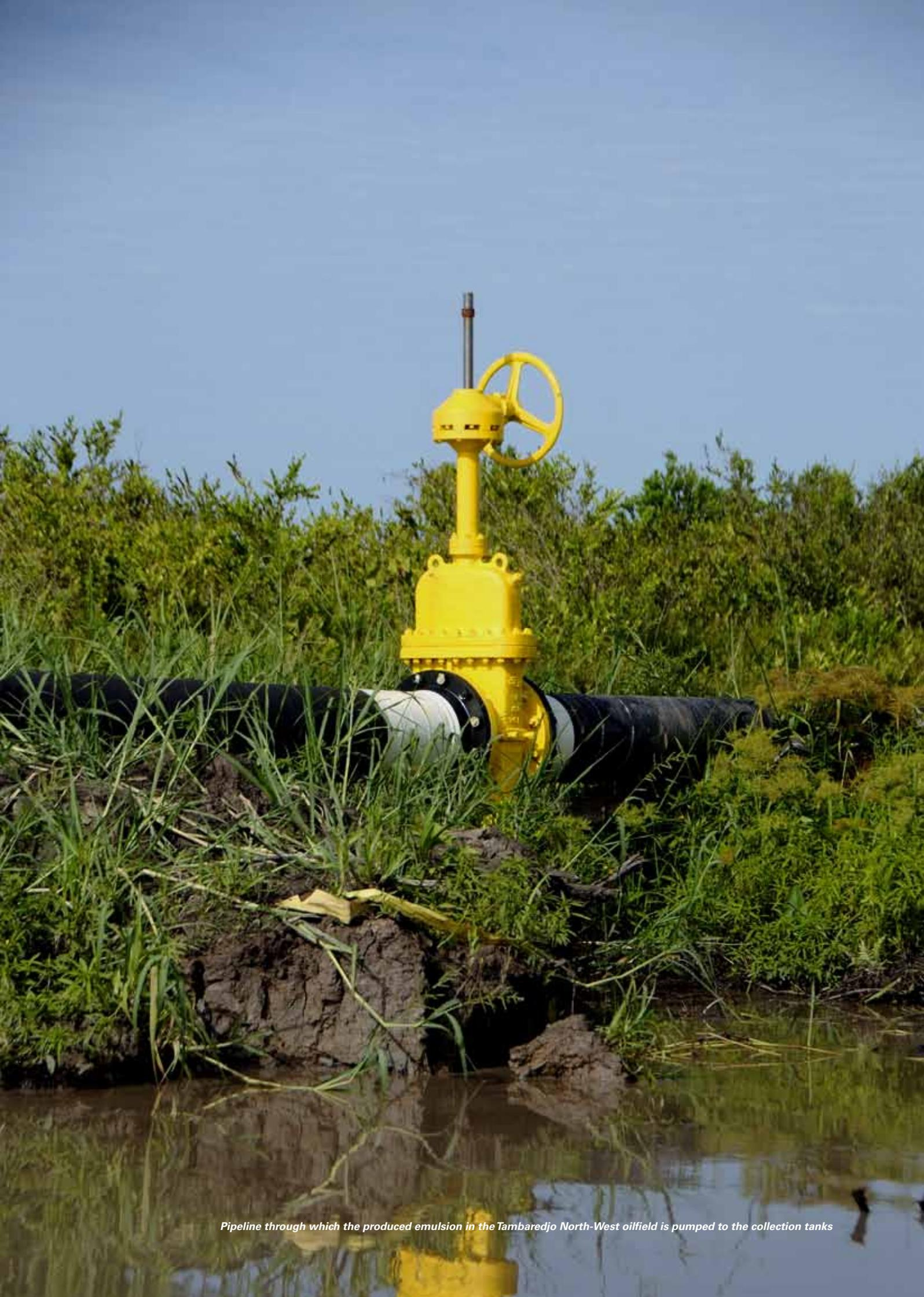
*Pipeline through which the produced emulsion in the Tambaredjo North-West oilfield is pumped to the collection tanks*
